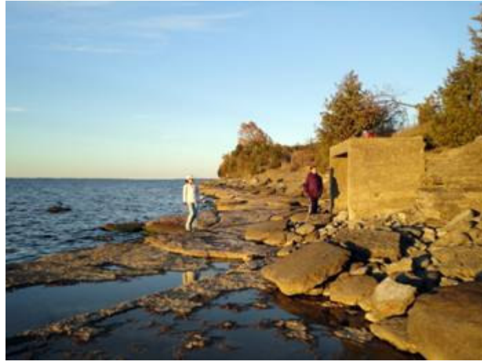
The pill box at Wehle State Park.
